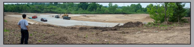
The storm drain and two detention ponds are complete. Cut and fill is about about 85% completion. A sewage line will run from town's connection point to the Islamic Community Center pad. The Water pipes will be run from the property line up to the Islamic Community Center pad. Also two fire hydrants will be installed. The parking lot will soon have crushed stone and work will start on the Islamic Community Center slab. InshAallah
