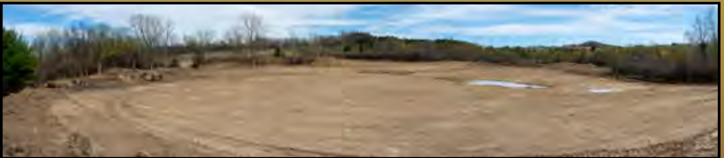
The cleared land for the Islamic Community Center
